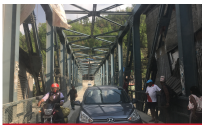
2 WAY BRIDGE, BUT ONLY ROOM FOR ONE CAR AT A TIME
