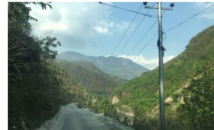
THIS ROAD GOES FROM KATHMANDU TO JIRI AND WAS BUILT BY SWITZERLAND OVER 20 YEARS AGO
