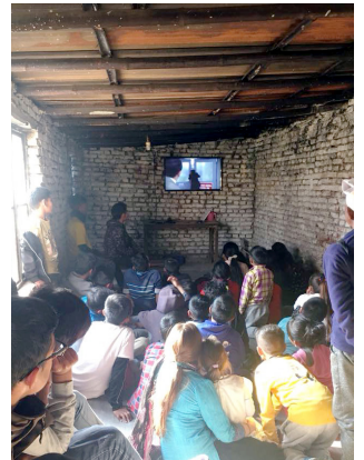
TV room before renovation
