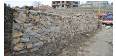
Finished with the wall!
