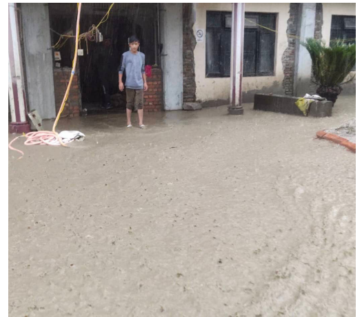
Water has moved to first floor, inside
