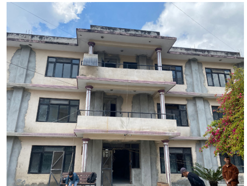
Almost ready after rooms and walls and plaster were done
